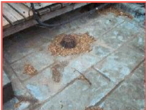
WATER DRAIN OUTLET
