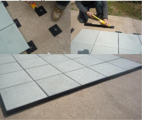
Guide to Laying Castle Promenade Slabs with Sikaflex on Aslon Paving Support Pads. This method will ensure that slabs are held in position when no edge restraint is available from upstands, walls, balustrades or the like.
